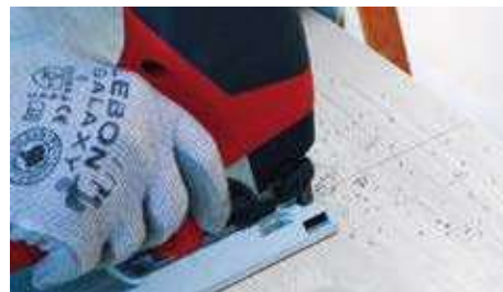
CUTTING WITH A SAW
